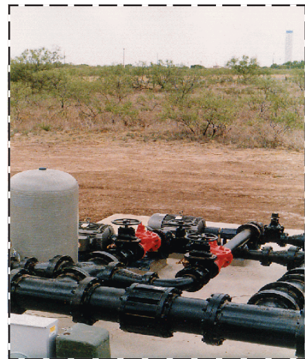
86 gallon tank replaces 30,000 gal standpipe
