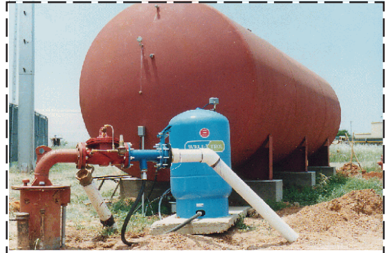
86 gallon tank replaces 10,000 gallon tank
