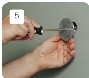
Tighten screw to secure anchor
