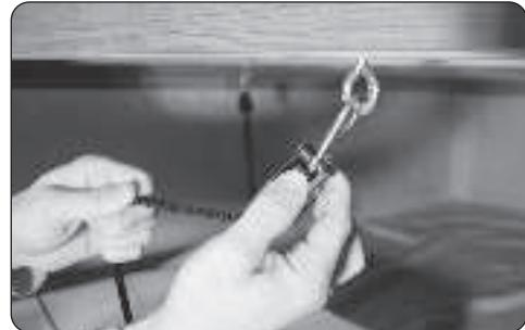
**Step 8:** Pull down on the ratchet rope, lifting the unit in place. We recommend pulling down on each individual ratchet rope 6-12 inches at a time until level.
