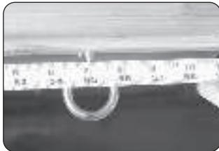
**Step 5:** Skip a joist to place the remaining two eye bolts on the joist parallel to the joist used for the first two eye bolts; leaving one joist not used between the two joists. Eye up the location of the remaining two eye bolts and position them straight across from the first two eye bolts used in steps 3 and 4. The placement should be close but does not need to be precise. Be sure to distance the two eye bolts 55" apart.
