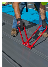
FSHS2 Works on 2" vertical seams with 13/16" width
