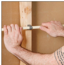
Push pipe to secure and lock
