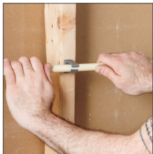
Place pipe into clamp
