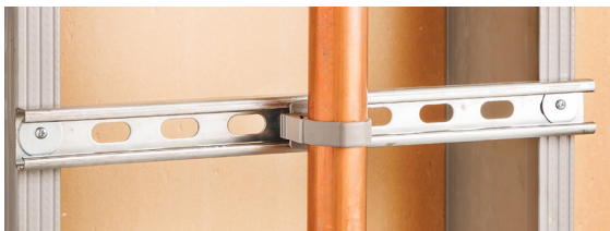
Showing Universal Strut Adaptor
