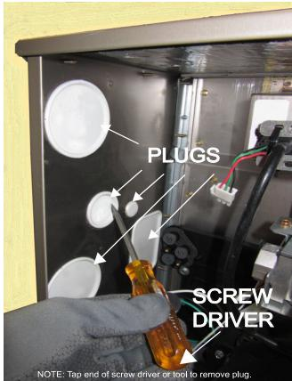
**NOTE:** Locate the plug that needs to be removed. Using a screw driver or tool, place end against rim on plug. Tap on the butt end of screwdriver or other tool to remove plug.
