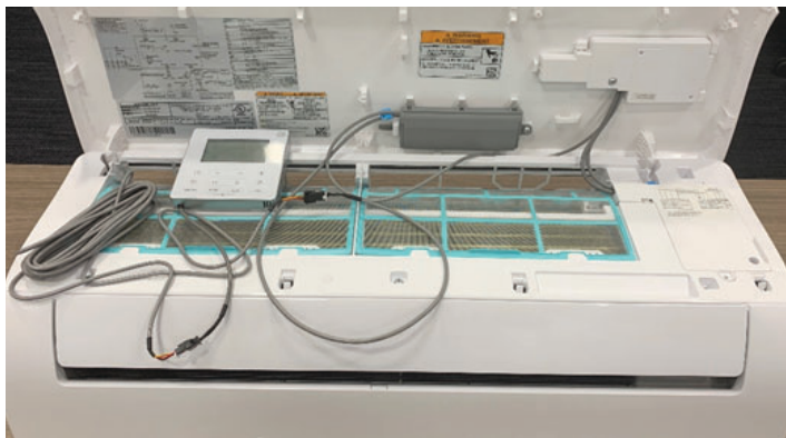
Fig. 16 — Close all the covers and install the extension harness
