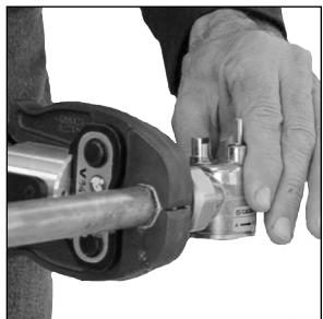
Check that the proper clamping jaws are installed and open jaw arms to set. Place jaw around valve end and double check proper insertion depth, press fitting.
